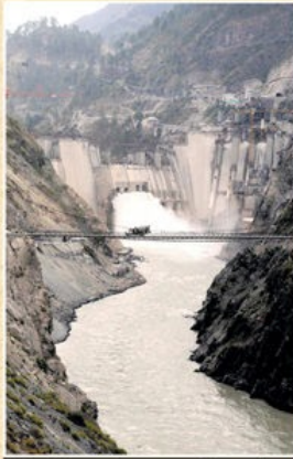
Baglihar dam on Chenab
