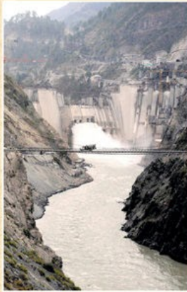
Baglihar dam on Chenab
