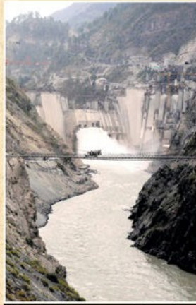
Baglihar dam on Chenab
